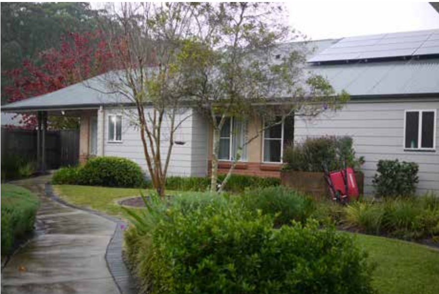
Solar panels on a rooftop
